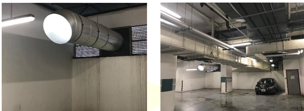
Daylight suntubes installed at Shun Lee Disciplined Services Quarters
