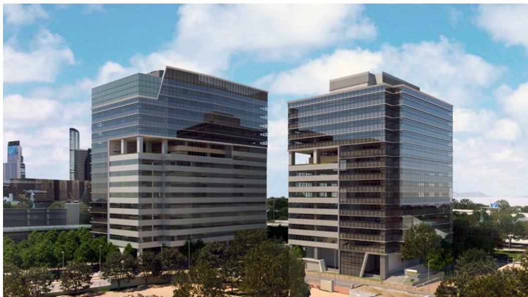
WKGO under development
