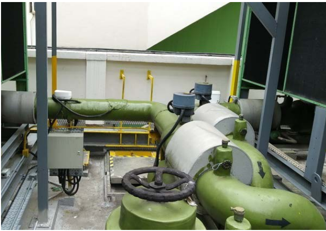
Replacement of flow meter and CCMS software to enhance the efficiency of chiller plants in Tai Po Government Offices
