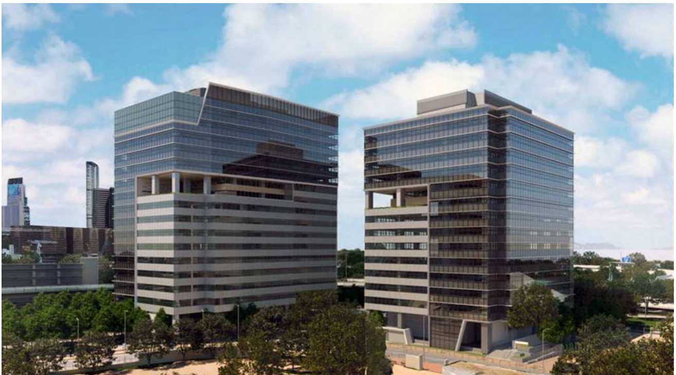
WKGO near completion
