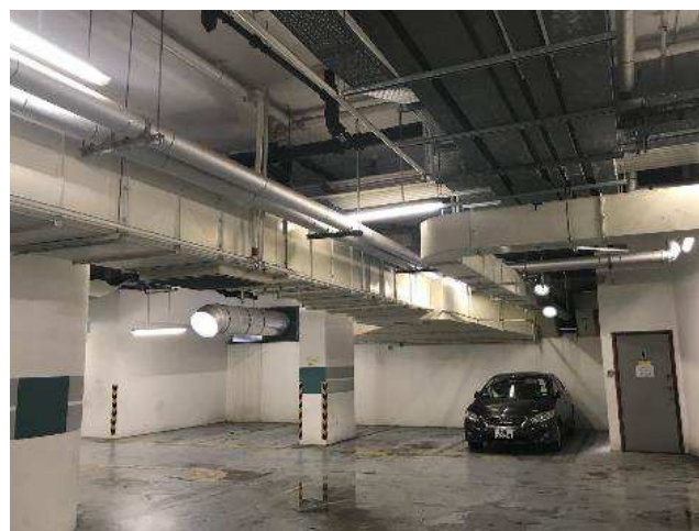
Daylight suntube installed at Shun Lee Disciplined Services Quarters
