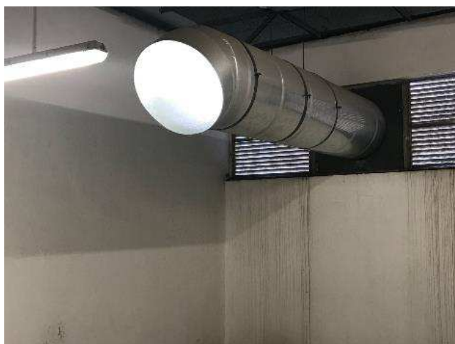
Daylight suntube installed at Shun Lee Disciplined Services Quarters
