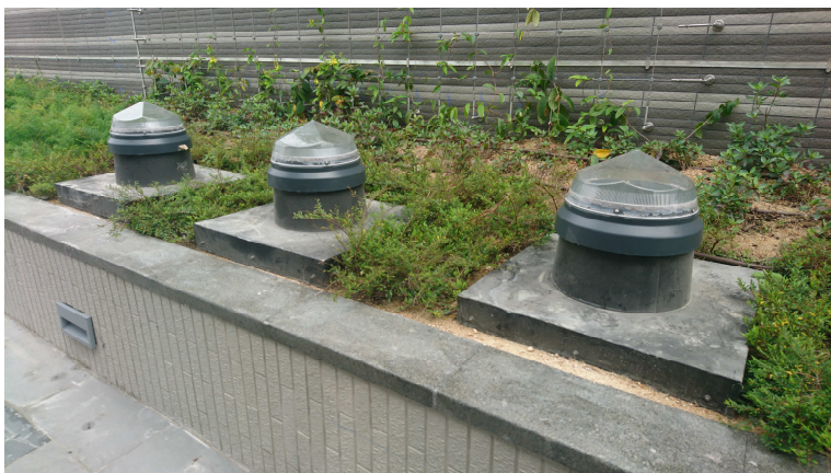
Daylight suntubes at WKGO
