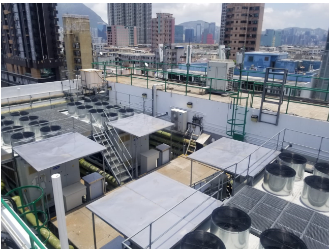
Replacement of air-cooled chillers and chilled water pumps at Tokwawan Government Offices
