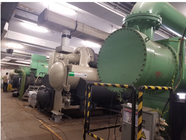
Replacement of sea water cooled chiller at Queensway Government Offices
