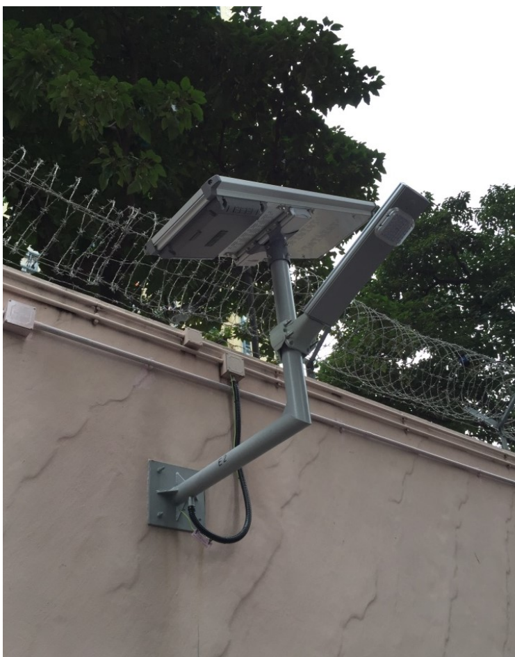
PV powered LED lamp at Kwai Fuk Court(left) and Aurora(right)
