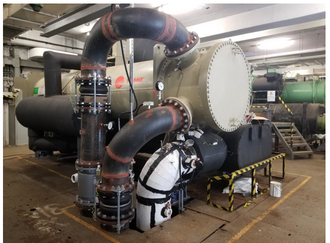
Replacement of sea water cooled chiller at Queensway Government Offices
