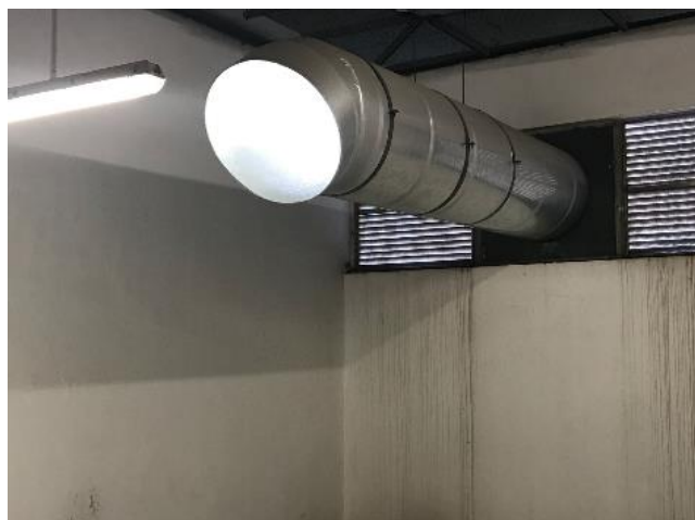
Daylight suntube at Shun Lee Disciplined Services Quarters
