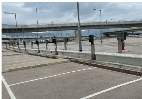
EV chargers at HZMB HKP car park
