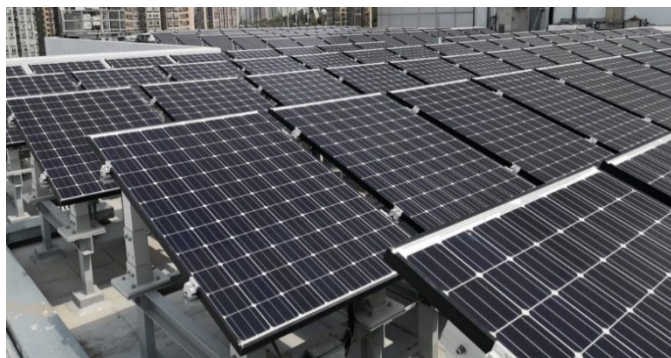
PV Panels at Tuen Mun Government Offices
