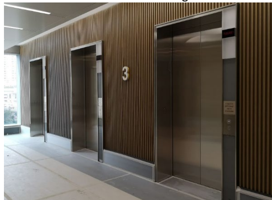
Power regenerative lifts
