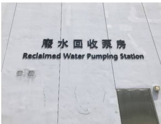
Reclaimed water pumping station in HZMB HKP
