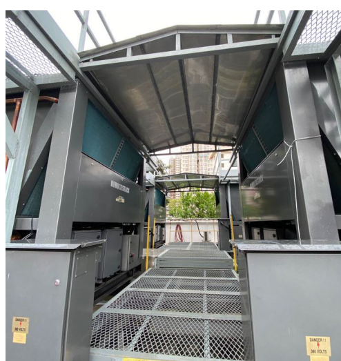
Replacement of air-cooled chillers and chilled water pumps with VSD at Tai Po Government Offices
