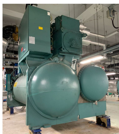
Seawater-cooled chiller at HZMB HKP
