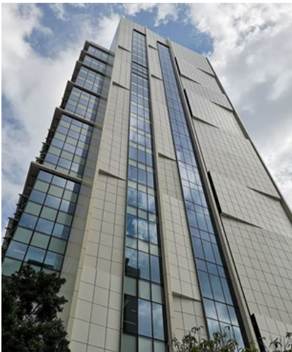
Solid wall of end-core
