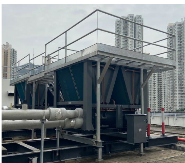
Replacement of air-cooled chillers with variable speed drive (VSD) at Tai Hing Government Offices
