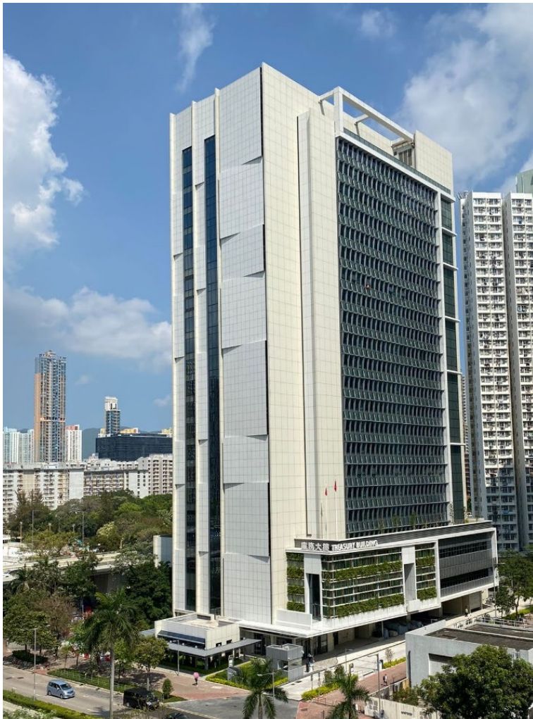
The Treasury Building is a new JUB project in Cheung Sha Wan.
