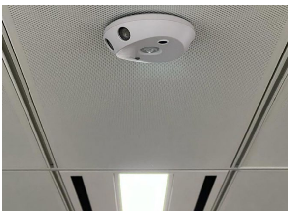
Occupancy sensor for lighting control at WKGO
