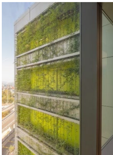
Vertical greening at WKGO
