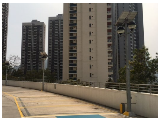
PV powered LED lamps at Aurizon
