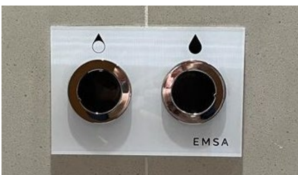
Dual flush toilet cisterns in Hong Kong-Zhuhai-Macao Bridge Hong Kong Port
