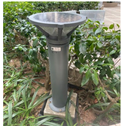
Solar bollards at Shun Lee Disciplined Services Quarters
