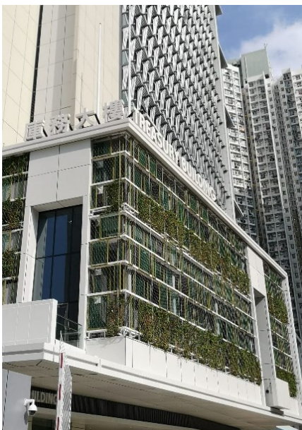
Vertical greening at Treasury Building
