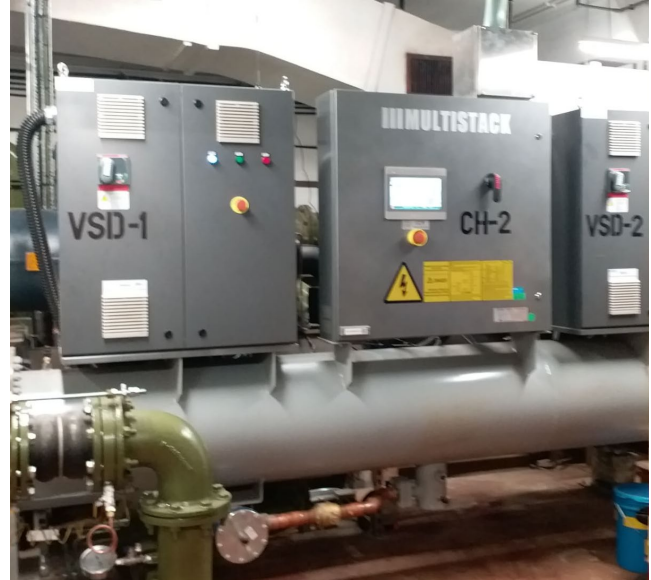
Direct seawater-cooled chiller replacement works at Kowloon Government Offices
