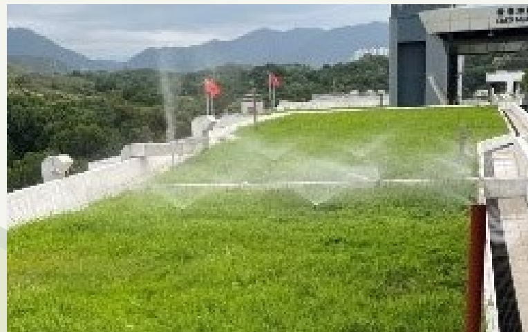
Irrigation by rainwater harvesting system at HYW BCP
