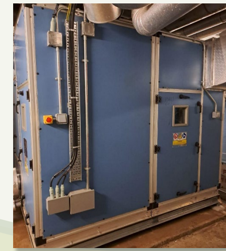
Replacement of primary air handling units at Ho Man Tin Government Offices
