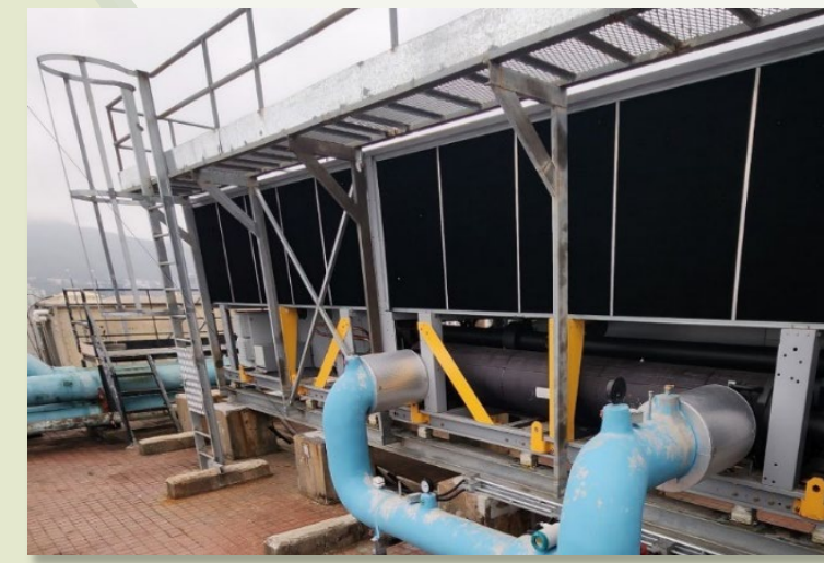
Replacement of air-cooled chiller at Wu Chung House
