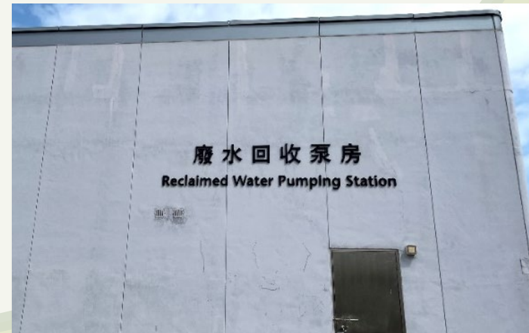
Reclaimed water pumping station at HZMB HKP
