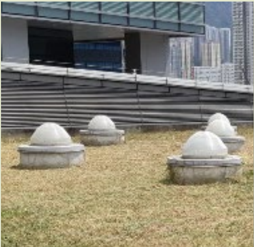
Light pipes at Trade and Industry Tower
