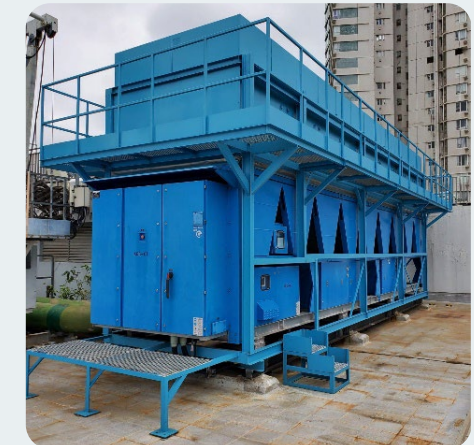
Replacement of air-cooled chiller at Eastern Law Courts Building
