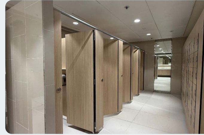
MiC construction for toilets at Tseung Kwan O Government Offices
