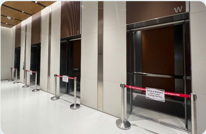
Suspending lifts during non-peak hours at Tseung Kwan O Government Offices
