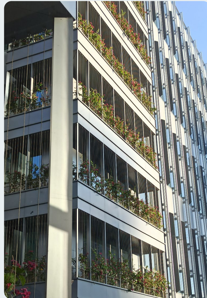
Vertical greening at Tseung Kwan O Government Offices
