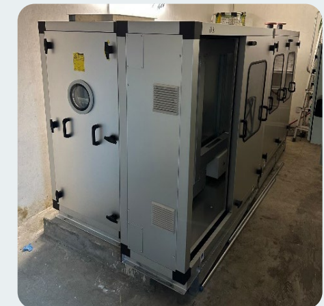
Replacement of air handling units at Wang Cheong Building
