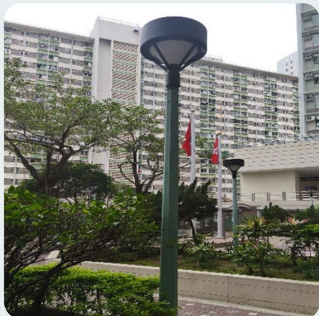
Solar lamp poles at Kwai Yung Court
