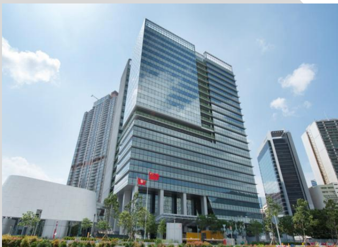
Joint-user Office Buildings
