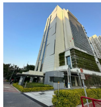
Joint-user Office Buildings
