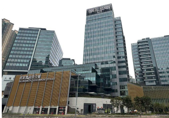
Joint-user general office buildings
